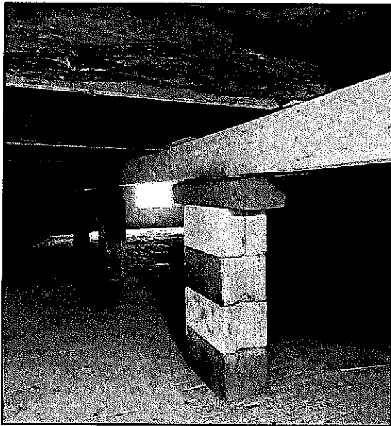
Figure 27: First floor structure, showing columns, centre beam, and joists
