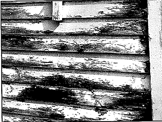
Figure 4: South face paint detail
