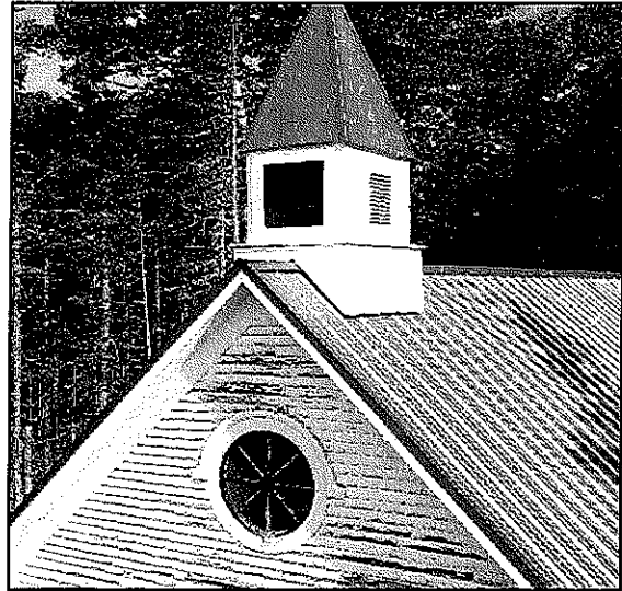
Figure 22: New metal roof with bell tower at south end
