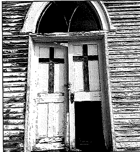
Figure 5: Entrance door damage
