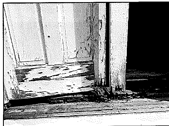
Figure 21: Deterioration on threshold and bottom of door
