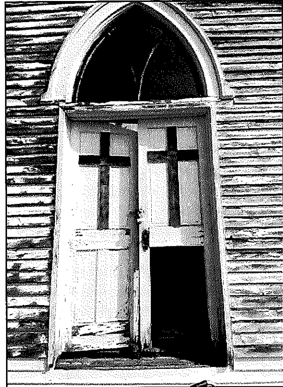
Figure 20: Missing door panel
