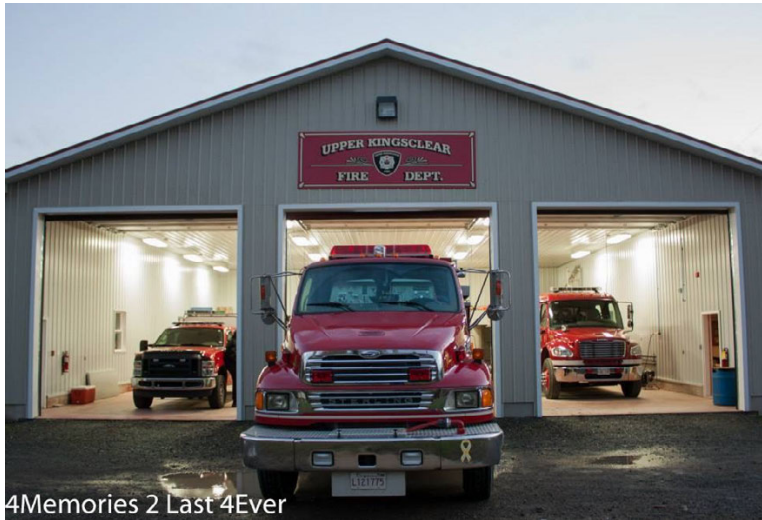
Expansion Completed at Station 1
